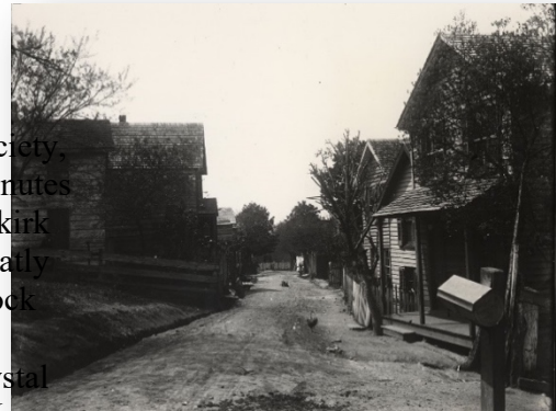
Figure 1. Queen City, a historically African American enclave located in what is now Crystal City, was destroyed by eminent domain to build the area around the Pentagon.
