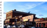
Figure 4. Independent retail operated by local residents are cornerstone to building and sustaining a vibrant community.
